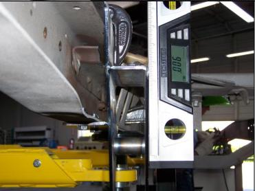
We need to make sure the brackets are square to each other and are sitting vertical before drilling any holes.
